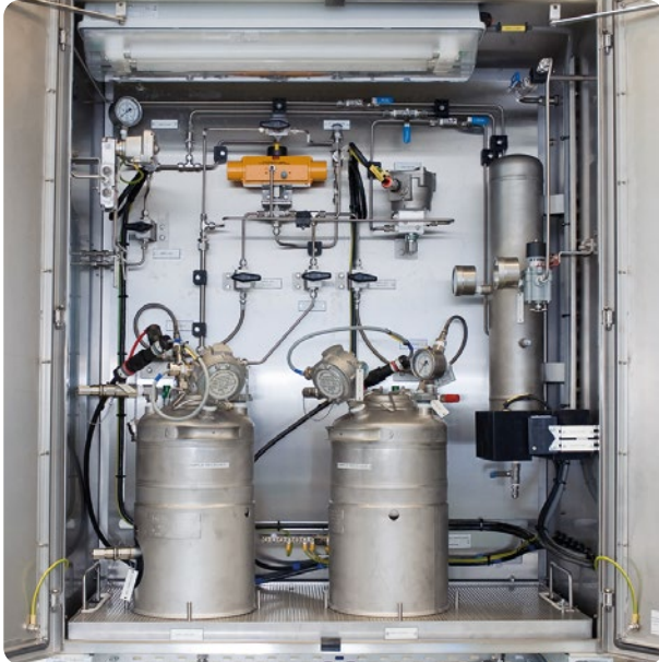
Example of an Automatic Crude Oil Sampling System comprising of a stainless-steel enclosure with heater, grab sample pump, bypass vanishing chamber sampler and an auto switchover mechanism to switch between the duty and standby sample container. A stationary mixing bench for mixing contents of sample containers was also part of the scope of supply.
