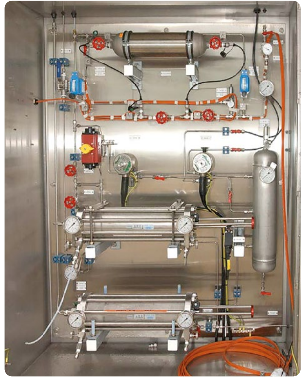
Example of a grab sampling system for flow proportional low temperature (-40/-50 °C) propane/butane sampling including take-off probe and bottle racks for precharge gasses. The LPG sampling system was supplied as part of a liquid metering package.
